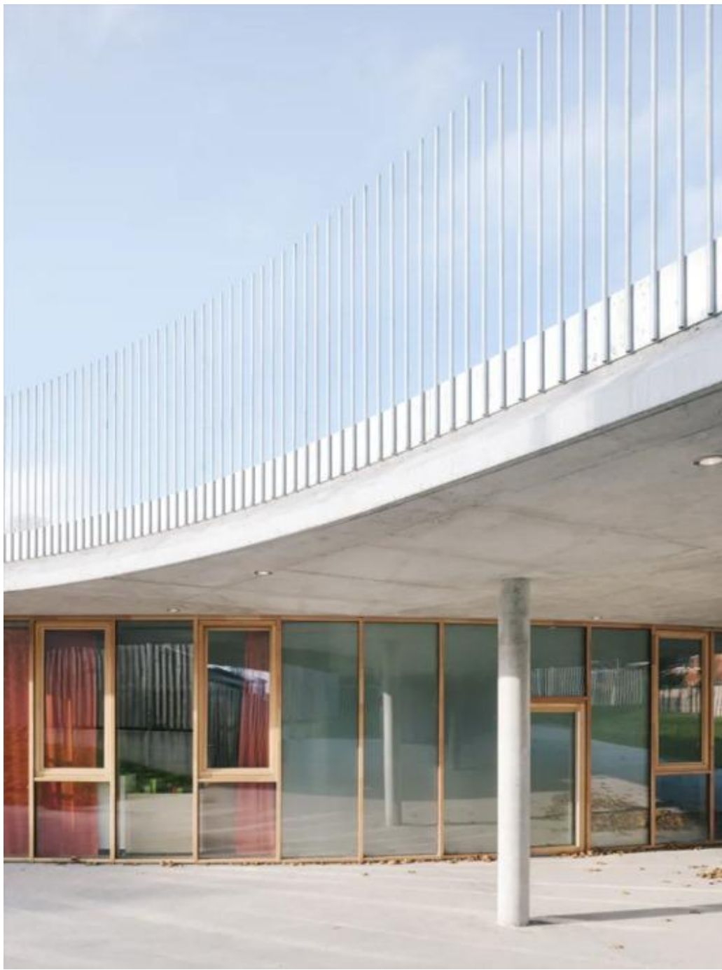
BAL - BALUSTRADE CONCRETE SLAB & GALVANISED BALUSTRADE
