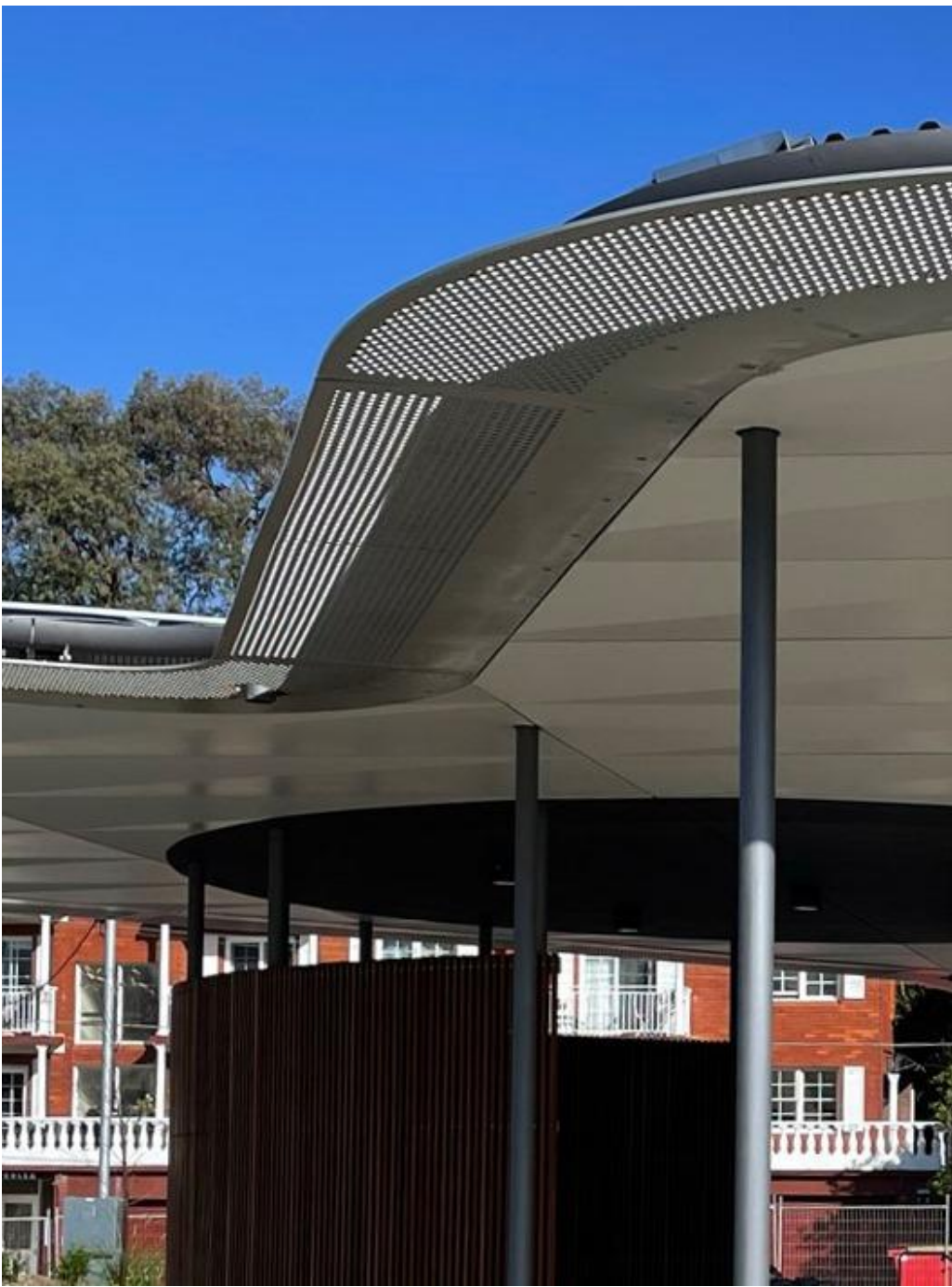
MF - METAL FASCIA TO AWNING ROOF CURVED METAL AWNING WITH STEEL FASCIA AND ROUND COLUMNS
