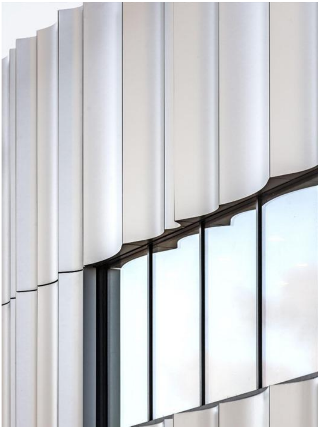
MCV - METAL CLADDING CURVED PANELS FACADE DETAILS, CURVED CLADDING ABOVE AND BELOW WINDOWS
