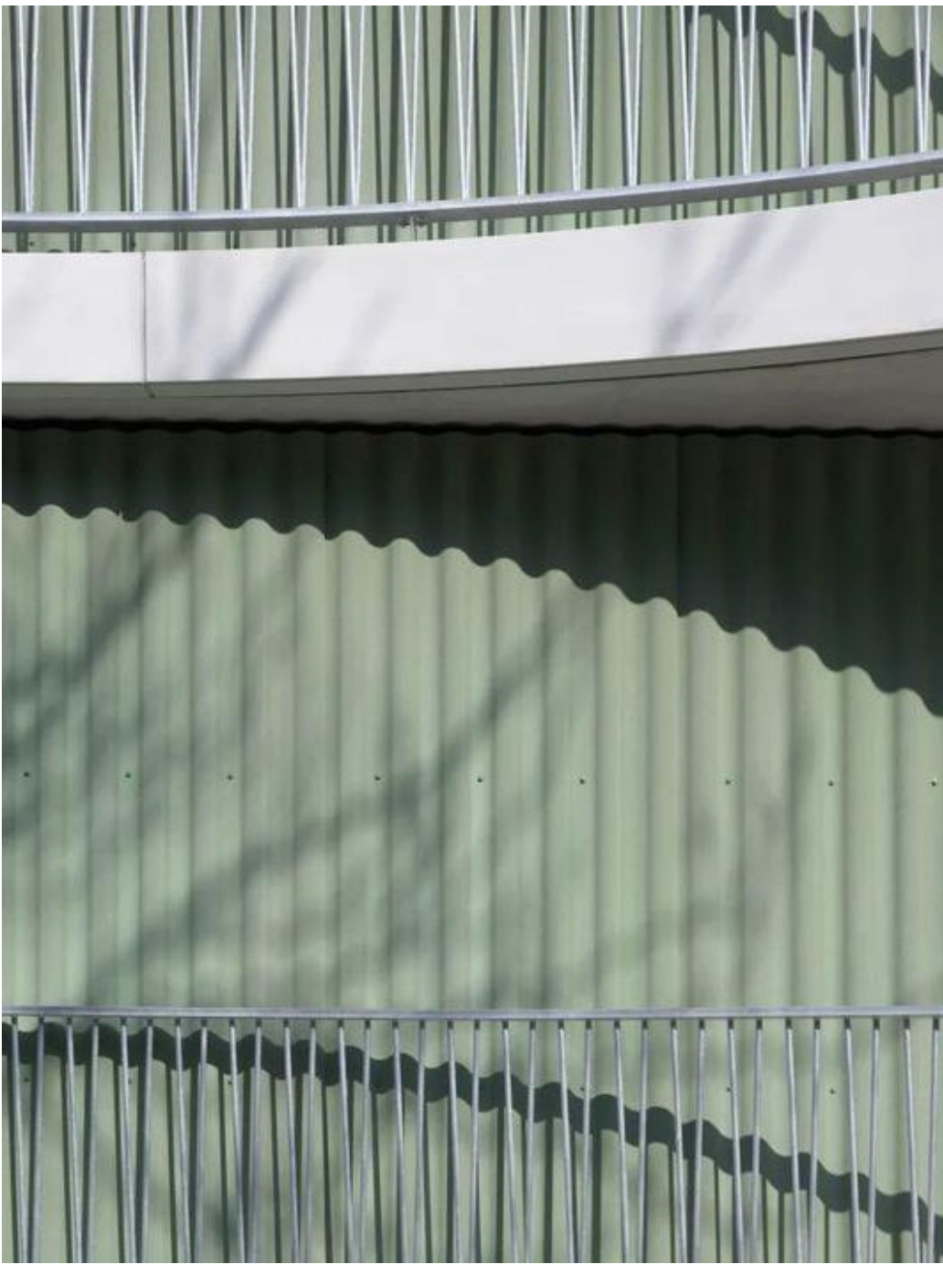
MC - METAL CLADDING WINDOW BOXES AND SUNSHADES POWDERCOATED IN PALE EUCALYPT
